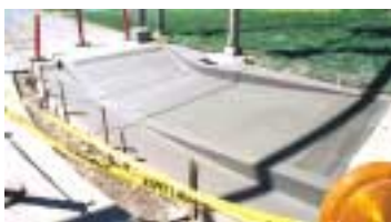
Measure A Entities continue to reconfigure street curbs for improved wheelchair access
