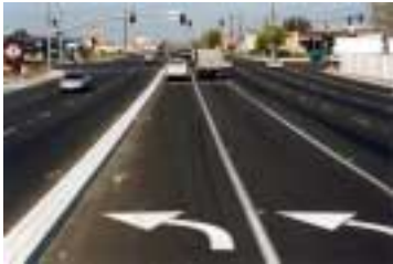
Intersection improvements at Elkhorn Blvd. and Watt Avenue included widened shoulders, dedicated right-turn lanes, new traffic signals and street signs, bicycle lanes, and double left-turn lanes (below)
