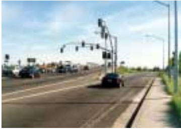
Interchange improvements at US Highway 50 at Bradshaw Road
