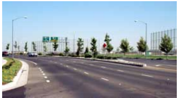
Looking north at the new extension of Truxel Road from San Juan Avenue to Interstate 80
