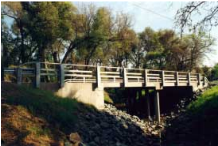
Replacement bridge on Woodside Drive west of Sylvan Road. Other bridge projects in the County's Highway Bridge Replacement and Rehabilitation Program are: Alta Mesa Road and Dry Creek (completed), Franklin Blvd. and the Mokelumne River (underway), and Bradshaw Road at Morrison Creek (underway).
