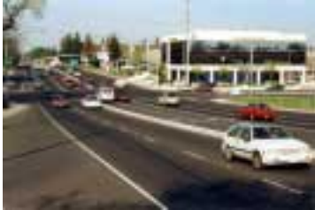
Intersection improvements at Elkhorn Blvd. and Watt Avenue included widened shoulders, dedicated right-turn lanes, new traffic signals and street signs, bicycle lanes, and double left-turn lanes (below)
