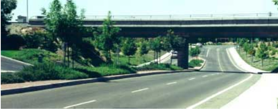
Looking westward at the recently-completed Exposition Blvd. extension project
