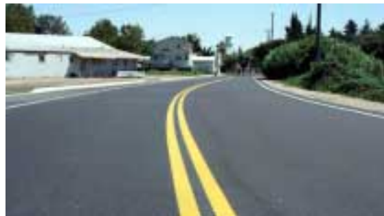
Isleton's Jackson Slough Road Reconstruction Project
