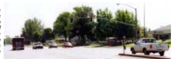
Work has begun on installing a computerized signal system on the South Natomas arterial system
